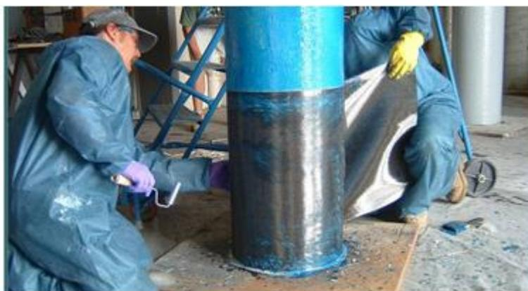
**Fig. 1.** Jacketing of FRP sheet around RC column
